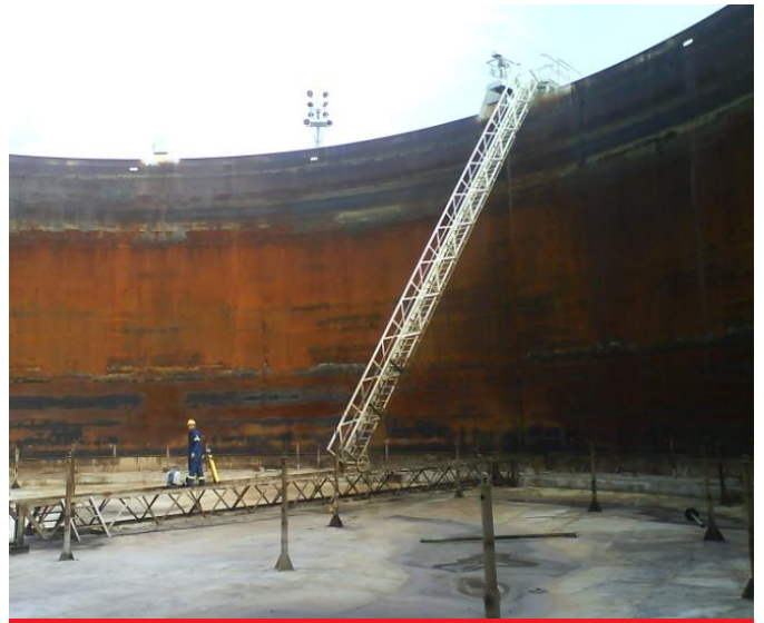
Cylindrical fuel tank interior
