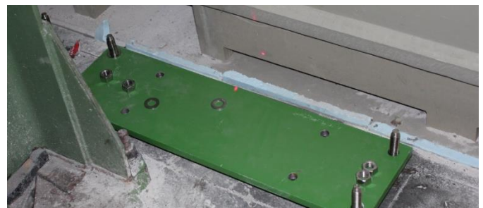
Squeeze rolls foundation plates on Main Clean Unit. The next step was the final alignment of the plate (orientation – position – height)
