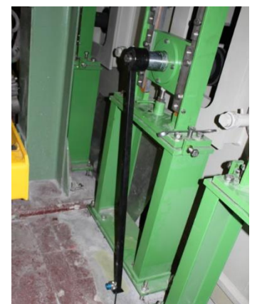
Squeeze rolls foundation plates on Main Clean Unit. The next step was the final alignment of the plate (orientation – position – height)
